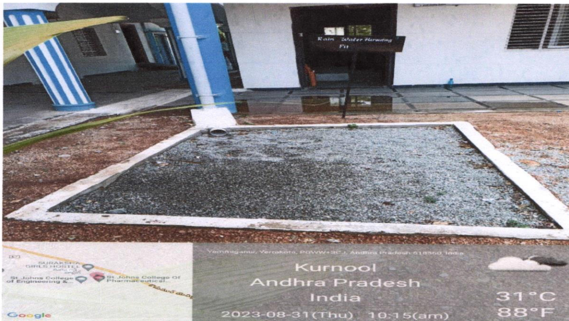
RAIN WATER HARVESTING PIT PHOTO
